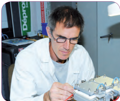
Simon Wood plumbing in the cooling circuit for the solid/liquid sample cells for FIGARO.
