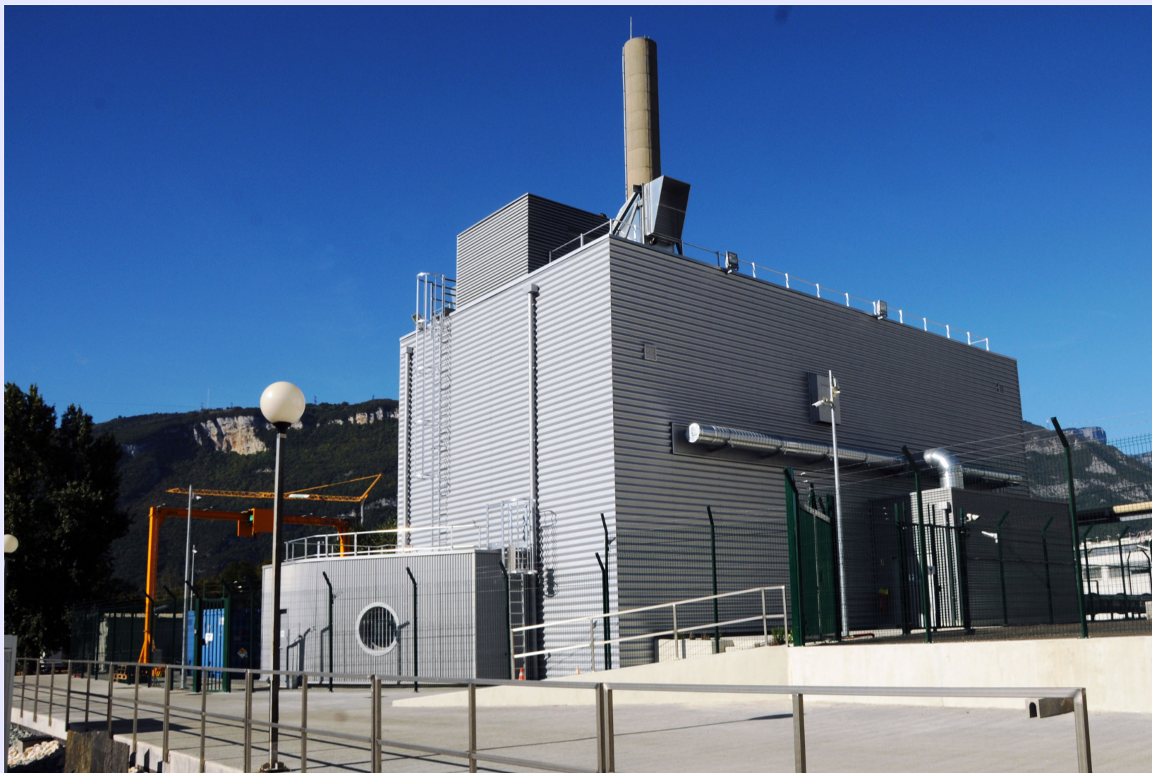
Fig. 11.7: The new highly reinforced building hosting both the heavy water treatment facility and, on the roof, the emergency control room PCS3.
