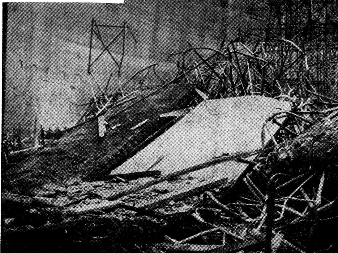
Fig. 5.5: Photograph of the future reactor hall after the collapse of a part of the roof under construction published 14 February 1970 in the regional newspaper Le Dauphiné Libéré .
