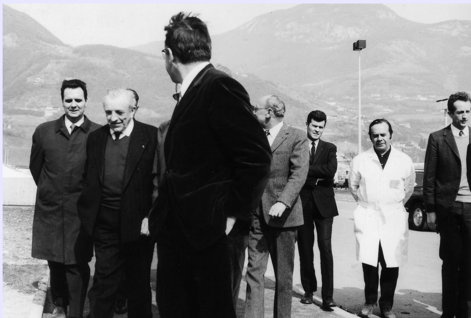
Fig. 5.4: Visit to the construction site in 1971 with Néel in the foreground, on his right Chatoux, and Droulers on the right edge of the picture.
