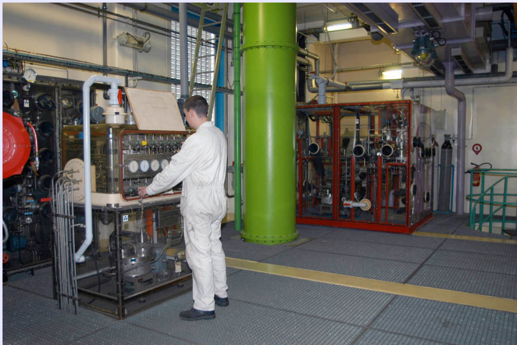
Fig. 5.7: The detritiation facility in 2004. On the left the monitor circuit and in the background the exhaust circuit for the tritium gas.
