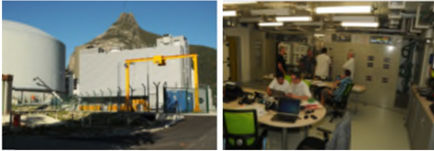
FIG.5. External view of new PCS3 (building) and emergency control
