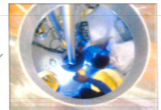
Nozzles-necks welding on the bottom of the machined lid
