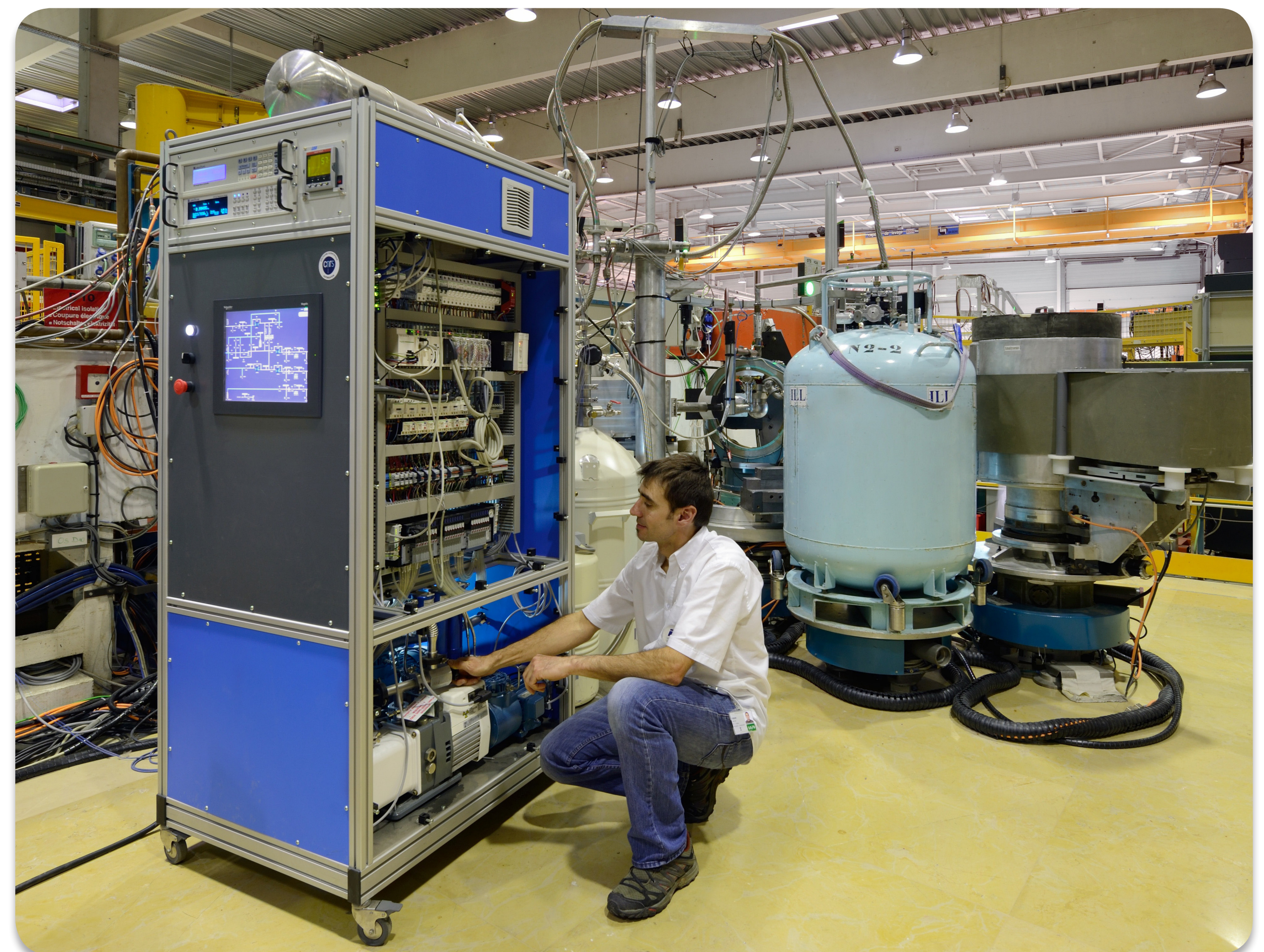
The complex automated gas-handling system of the closed-cycle dilution system on D10. © Ecliptique – Laurent Thion
