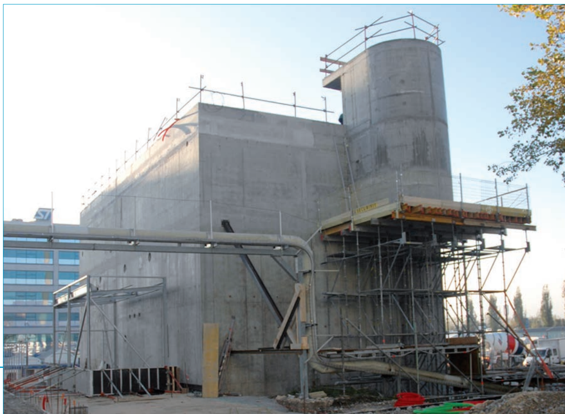
The new PCS3 control room in construction.
